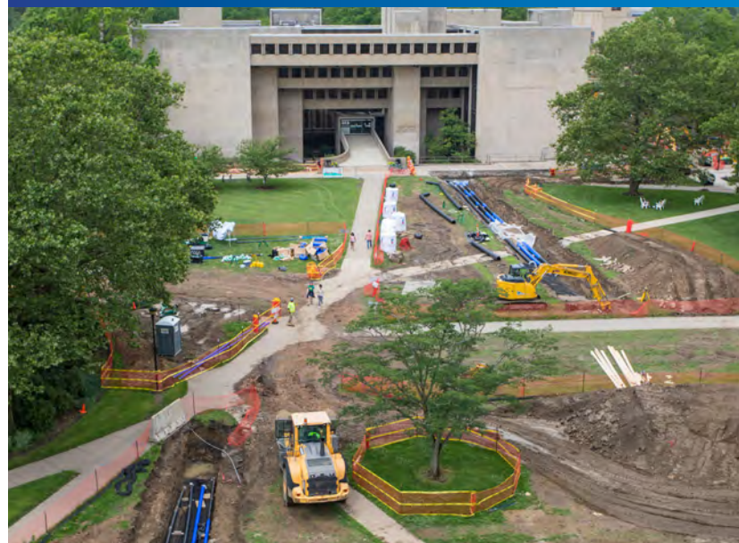
Aerial view of Oberlin College and Conservatory's new heating and cooling distribution piping, installed as part of the new carbon-free district energy system. Photo credit: Yvonne Gay Fowler
