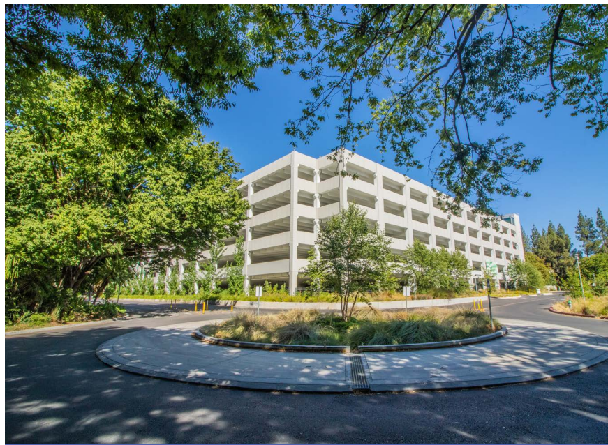
Dry well and Park Smart Gold Parking Structure 5 at Sac State. Photo credit: Sac State Sustainability
